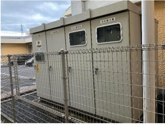
A photograph showing a row of three large, light-colored metal power conditioner cabinets. The cabinets are situated outdoors on a concrete pad. In the foreground, there is a silver metal chain-link fence. The background shows a clear sky and a portion of a building. |
